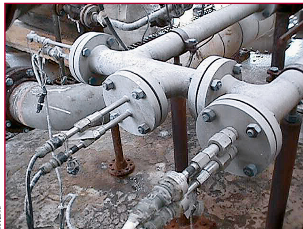
SwRI developed and implemented multi-electrode array sensor (MAS) probes to monitor localized corrosion of chemical process system components in real time.
