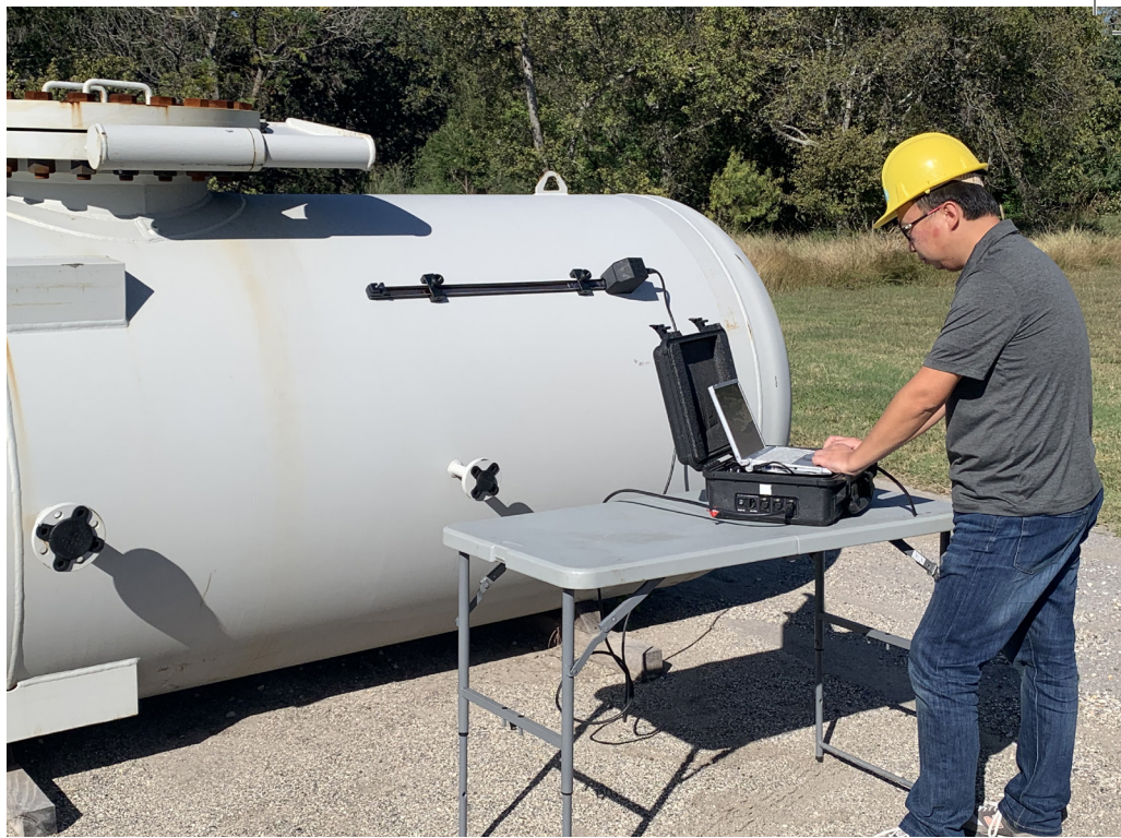
Probe attached to storage tank wall during guided wave screening of generalized corrosion area.
