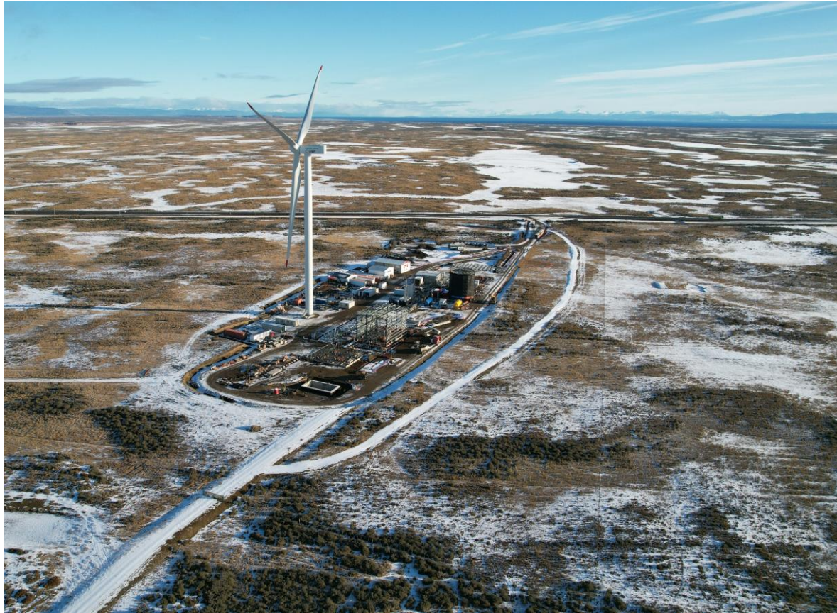
MAN Energy Solutions supports Porsche AG and HIF in its Haru Oni PtL project in Chile
