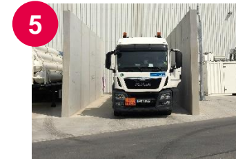
H2 filling station
