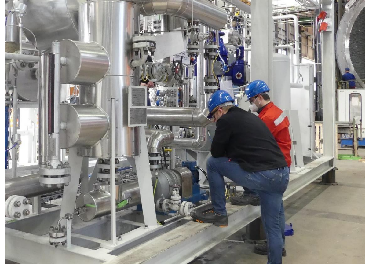
Methanol skid based on JM technology ready to ship
